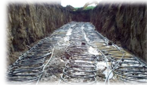
A horizontal closed loop heat sink.
